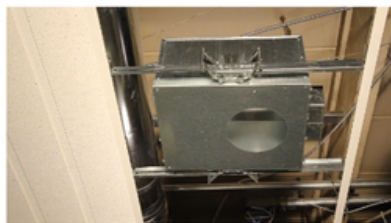
Fig. 70 Downlight suspension from T-bar
