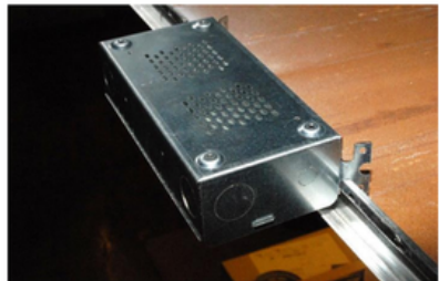
Fig. 49 Mounted to T-Bar using the integral T-Wings
