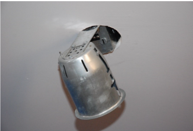
Fig. 7 Typical retrofit or remodeler assembly being rotated into hole in existing ceiling
