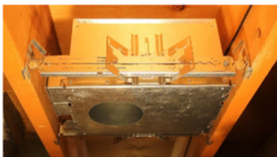
Fig. 69 Downlight suspension from wooden joists
