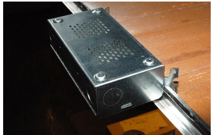
Mounted to T-Bar using the integral T-Wings
