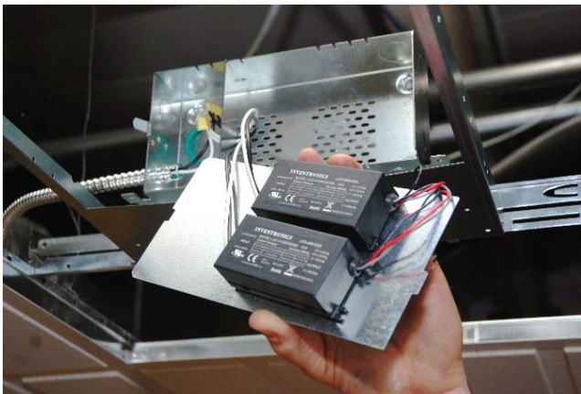
Mounted to Plaster frame with Drivers installed to cover
