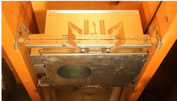
Fig. 52 Left: Downlight suspension from wooden joists, Right: from T-Bar
