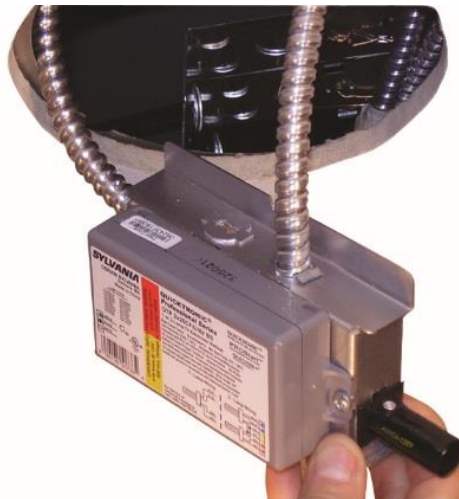
Fig. 35 Inner junction box cover (3D Cover #1242-18B) with mounted driver, removed for servicing below ceiling
