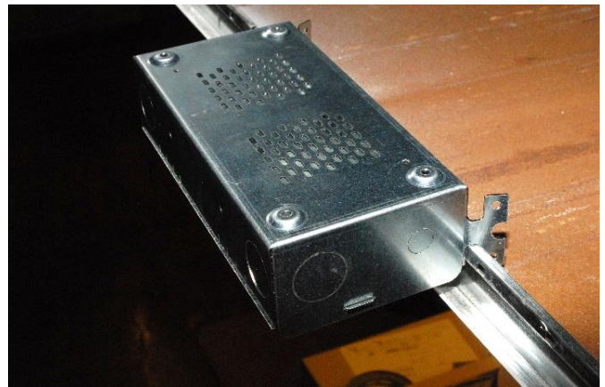
Mounted to T-Bar using the integral T-Wings
