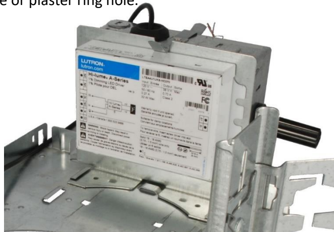
Fig. 37 Driver affixed to outside face of Inner junction box cover (1242-18), mounted to junction box 1232
