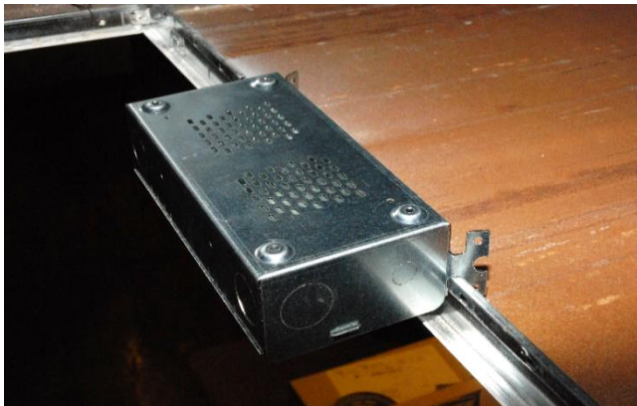
Fig 66: Mounted to Plaster frame with Drivers installed to cover
