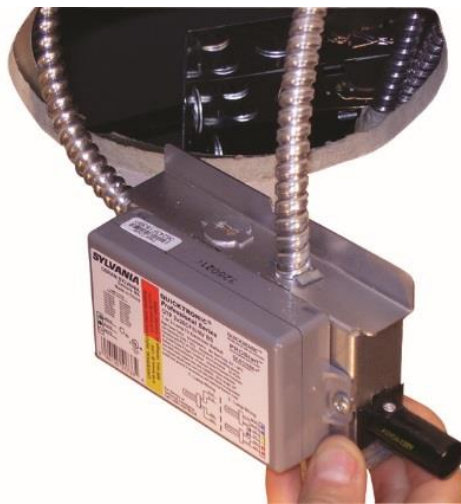
Fig. 38 Inner junction box cover (3D Cover #1242-18B) with mounted driver, removed for servicing below ceiling
