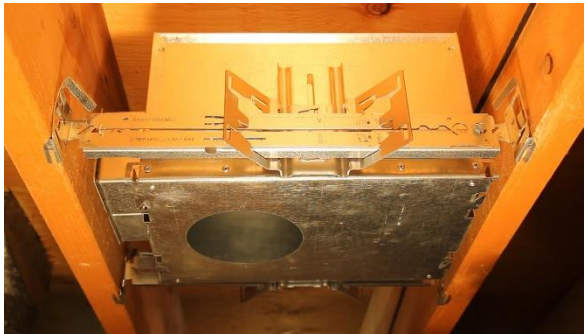
Fig. 57 Left: Downlight suspension from wooden joists, Right: from T-Bar
