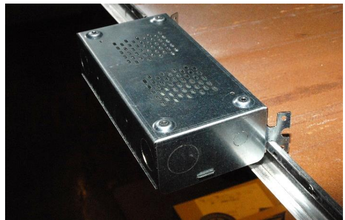
Mounted to T-Bar using the integral T-Wings
