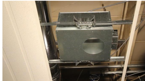
Fig. 57 Left: Downlight suspension from wooden joists, Right: from T-Bar
